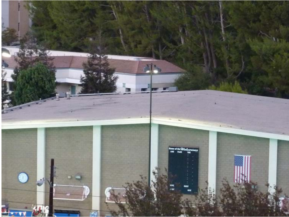
View from on top of the Development site looking at Taper Athletic Pavilion at before sunset
